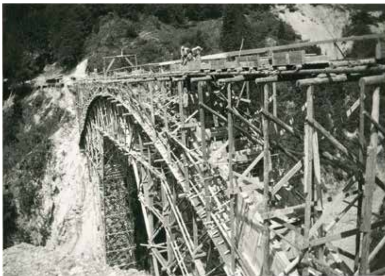
Figure 6: “Salginatobel Bridge at Schiers. Bh.: Graubünden canton”. Execution: Prader & Cie. AG, Zurich - Chur, centring: project and execu- tion R. Coray, Chur. 1929/30. Black-and-white print, rectangular (landscape format), 6.5 x 8.5 cm, ETH-Bibliothek Zurich, image archive (Hs_1085-1929-30-1-37).
